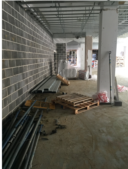
Enclosure of the new welding-shop
