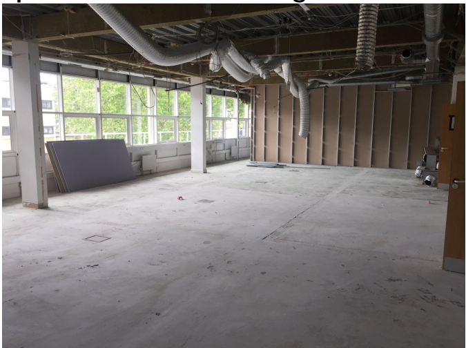
Space for the two new large classrooms
