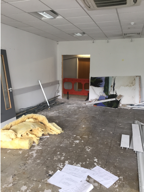
Retained classroom with the new opening to the corridor
